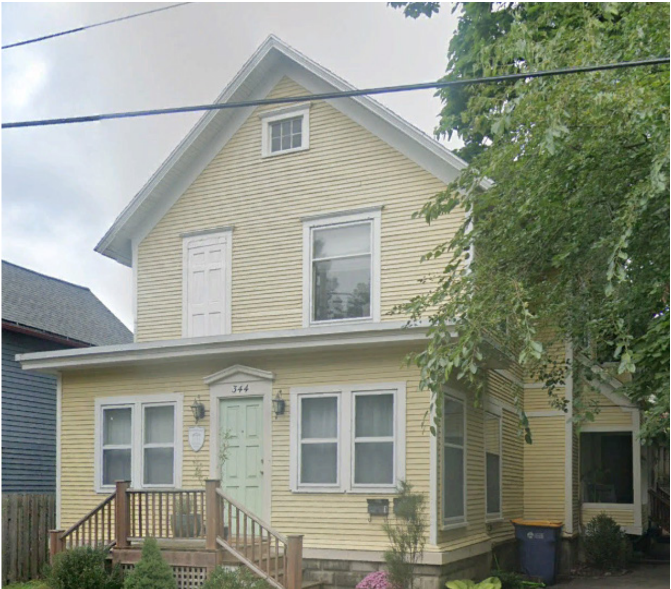
Duplex on Prospect Ave SE
