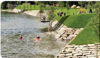
Design stacked, back-sloped limestone riprap to high water level. Steep mown slopes should be avoided unless higher maintenance is acceptable. Image: Bridgepark Müngsten Village; Wuppertal, Germany | Credit: Atelier LOIDL
