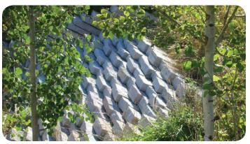
Stepped limestone riprap, poured-in-place, or sculpted concrete stone can be constructed as stepped wall.
