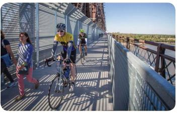
Example of a pedestrian/bike connection on an active railroad bridge. Design consists of a perforated steel deck with protected edge, set atop existing bridge footing. Big River Crossing; Memphis, TN | Image Credit: www.bigrivercrossing.com
