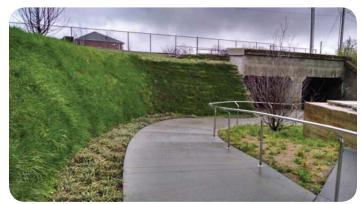
Reinforced earth green walls can be used in locations that are less susceptible to ice and flood damage. Image: Boneyard Creek Improvements; Urbana, IL | Credit: Wenk Associates
